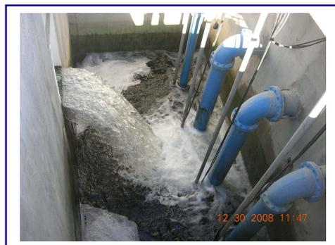
Figure 1: A plunging jet of wastewater into a wet well, entraining air at the pumps' intake
