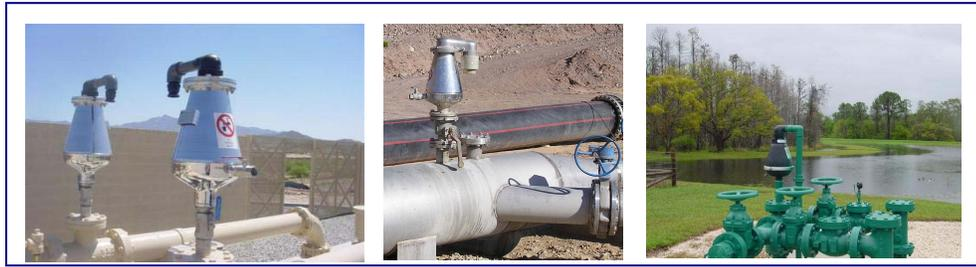
Figure 4: Stainless steel and composite material combination air valve for wastewater
